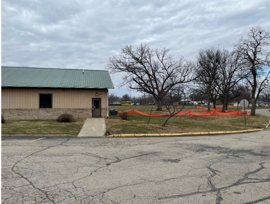
Figure A1: Front of the Dining Hall
