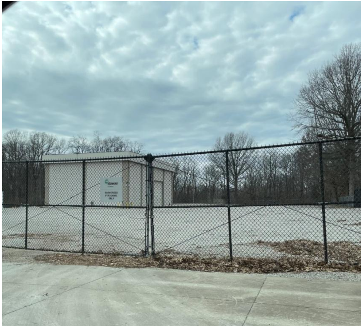
Figure A4: Fencing and Signage at Ameren CIPS Site
